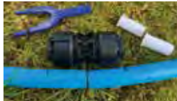
1 Cut pipe at leak. Mark pipe sections at width of joiner.
