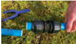
2 Insert pipe liners in pipe and slide joiner onto pipe over leak.
