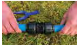
3 Position joiner so it is level with markings.
