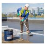
parapets, sky lights, ventilation pipes, metal supports and lightning protection rods are integrated in the surface waterproofing without any seams or joints.
