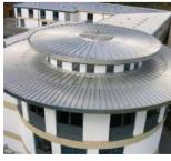
A superior quality raised standing seam roofing and cladding system that enhances aesthetics and provides a weather tight joint above rainwater flow. The perfect choice for an exceptionally wide range of new build, refurbishment roofing and vertical facade
