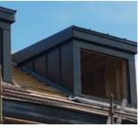
The Colorcoat Urban<sup>®</sup> standing seam system is designed for roofs and walls.
