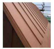
Renolit Alkordesign combines the aesthetic appearance of a metal standing seam (lead, zinc, copper or aluminium) with the benefits of a pliable synthetic roof through the application of a purpose made extruded profile.
