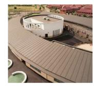
A calendered and laminated membrane of flexible PVC and polyester reinforcing for use in the Alkor mechanically fixed system. Mechanical fixing offers the benefits of less interruption during periods of inclement weather, a designed value for wind load and speed of installation.
