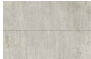
Cracked Cement (60cm x 30cm tile size)
