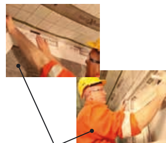
The Vario® membrane is sealed to masonry walls at ceiling level. Vario® Tape (in the above images, Vario® Bond) is used to seal the point where timber separating floors penetrate the outer blockwork and where windows meet blockwork.
