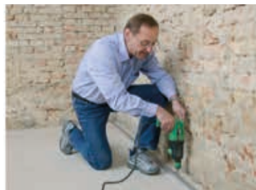
2. Secure Floor and Ceiling U-channel
