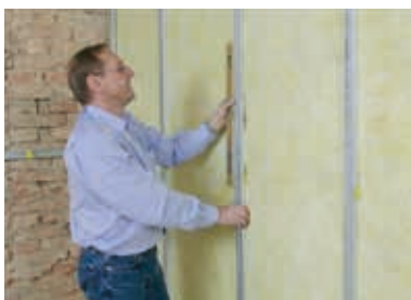
5. Fix plastic clip on vertical C-channel, adjust until plumb and lock in place
