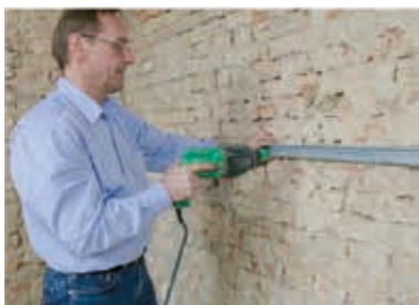
1. Secure 2.4m C-channel
