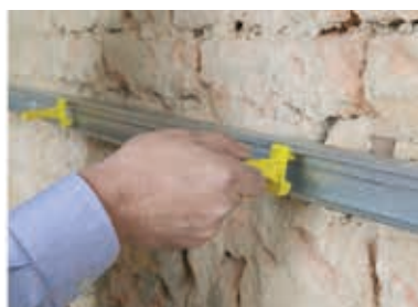
3. Fix plastic clip on horizontal C-channel
